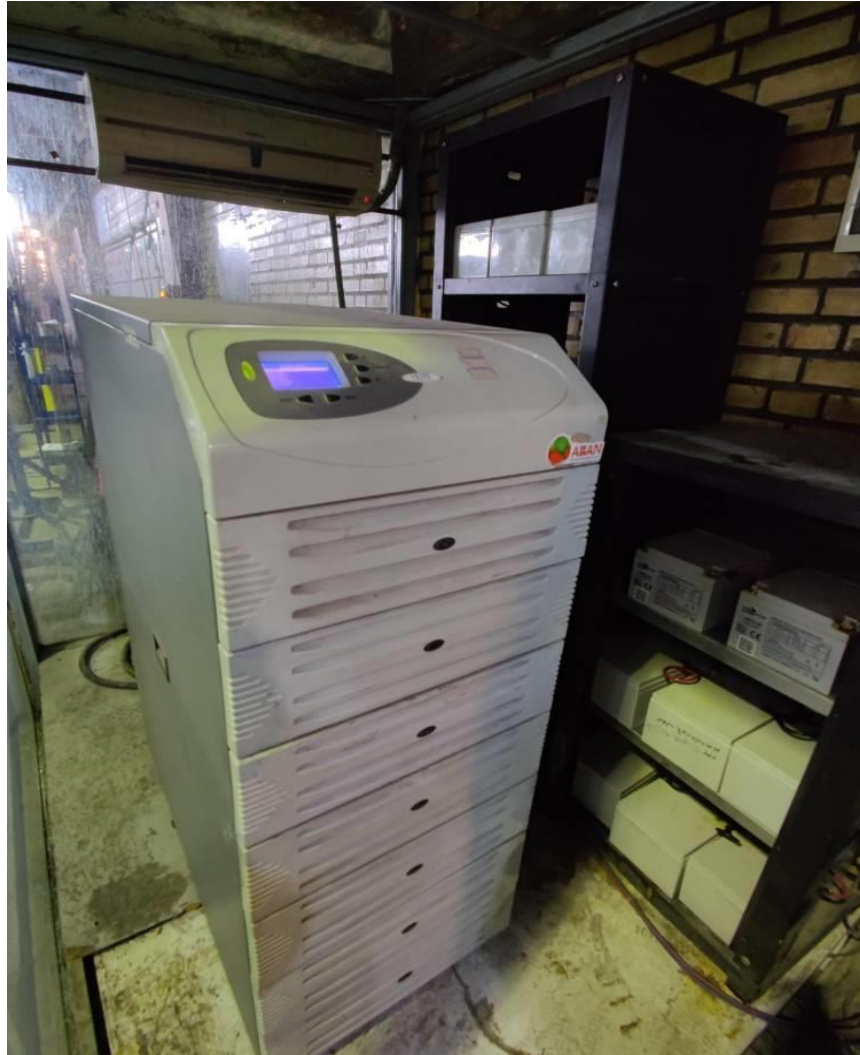
Fig. 5. A SCADA-communicating UPS system integrated with a tempering furnace
